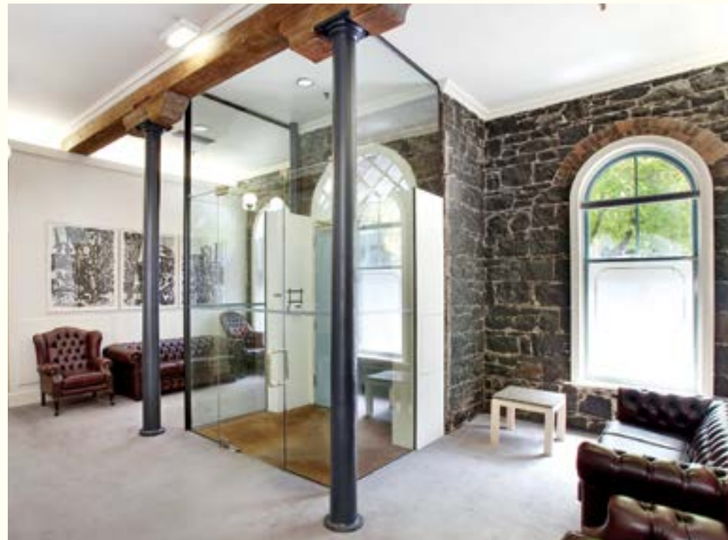
A private Trust of Barristers bought and renovated -573- in 1984. The ground floor had a reception area and individual legal chambers. Frank Knight STATE LIBRARY VICTORIA
