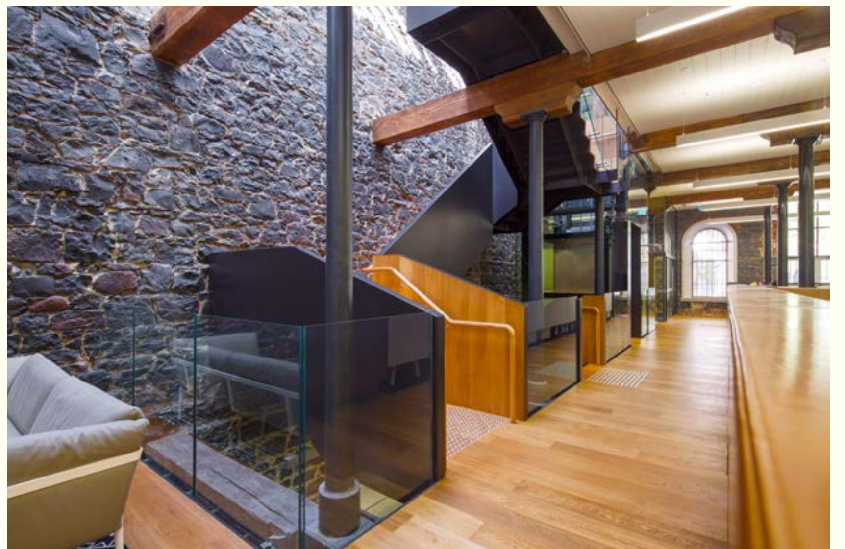
Meeting of old and new. The elegant open timbered modern internal structure is set against the strength and age of the original bluestone wall. JOHN WARDLE ARCHITECTS
