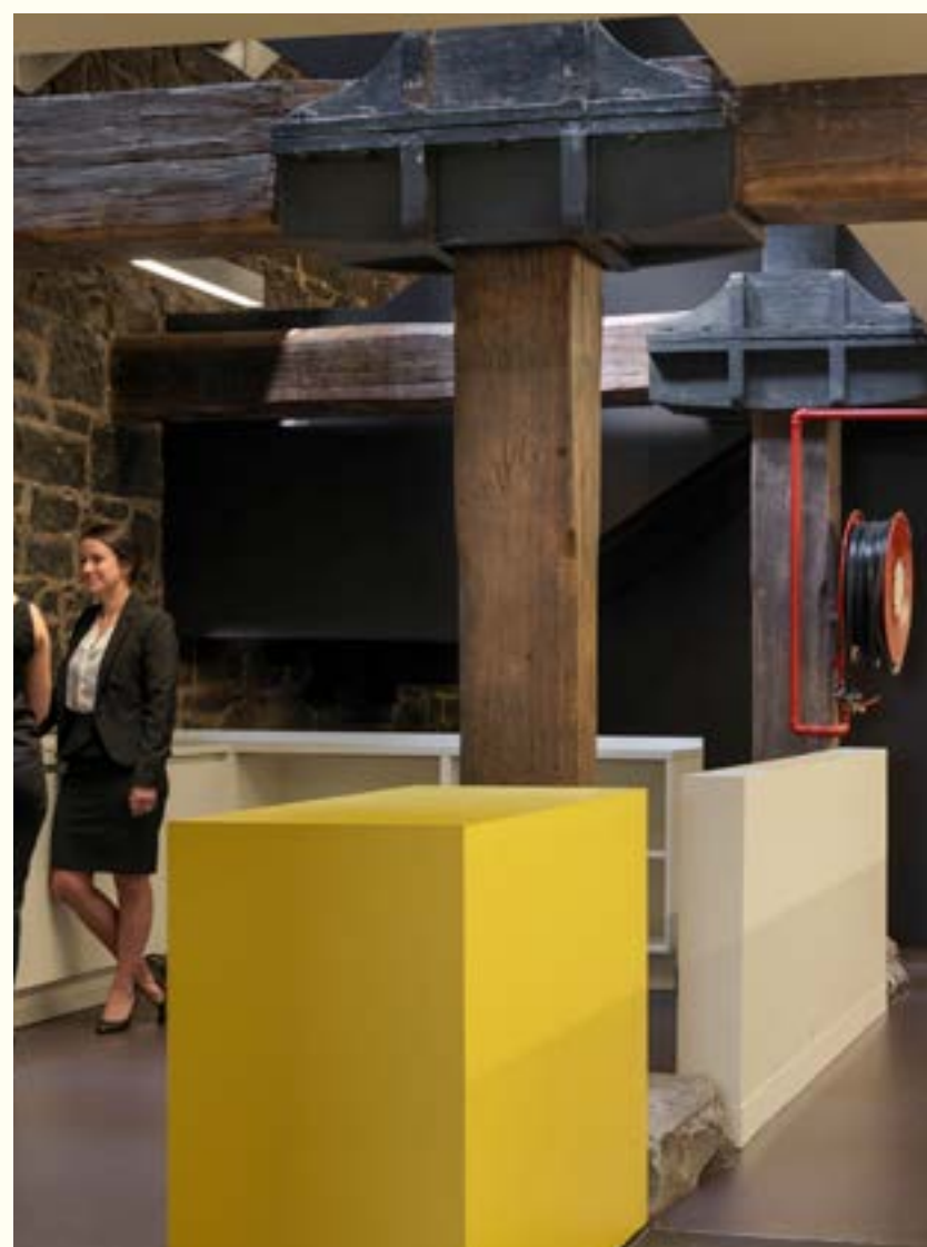
The industrial sized cast iron shoes encase the beams and pillars of refurbishment for Arnold Thomas & Becker Lawyers. JOHN WARDLE ARCHITECTS
