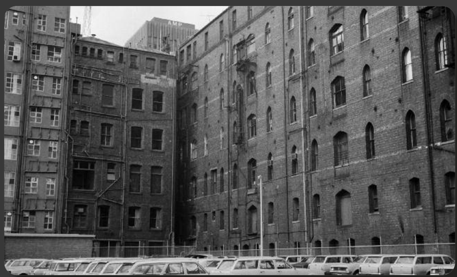
The rear of the Rialto building from Robbs Lane, 1969.
