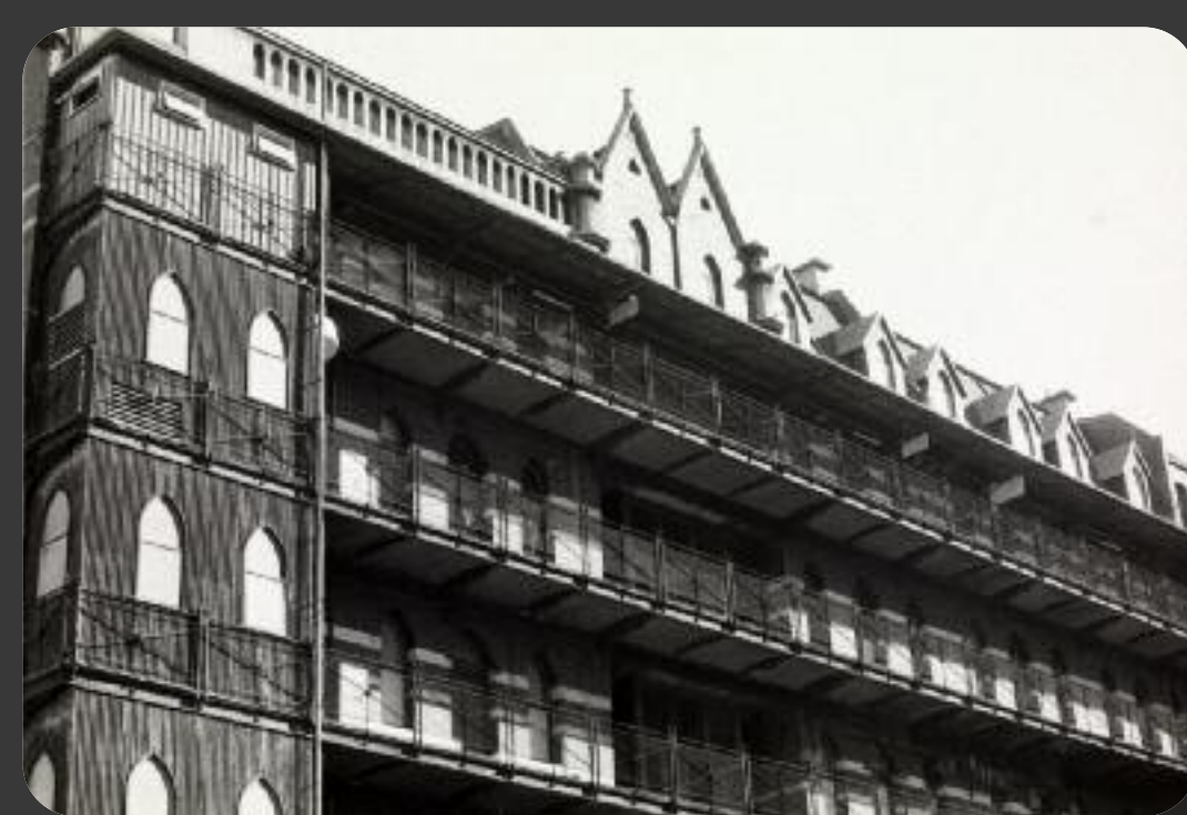
The rear of the Rialto building, view from Flinders Lane featuring the controversial iron urinals, 1977.
