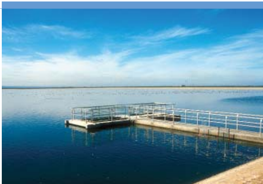
Stabilisation lagoons hold water from Bolivar Sewage Plant for approximately 20 days prior to treatment at the Recycled Water complex at Bolivar, north of Adelaide, South Australia. Image courtesy of ©CSIRO Land and Water
